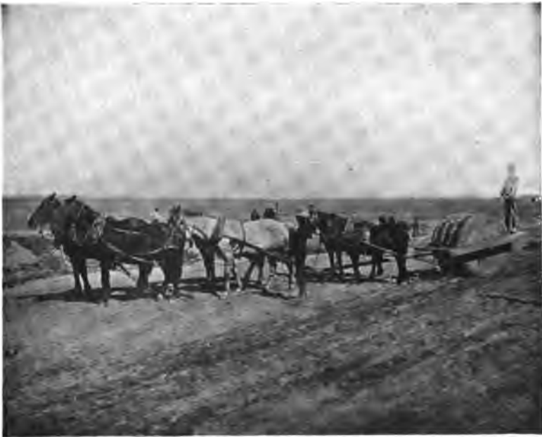
FIG. 205.—Grooved Concrete Roller.
